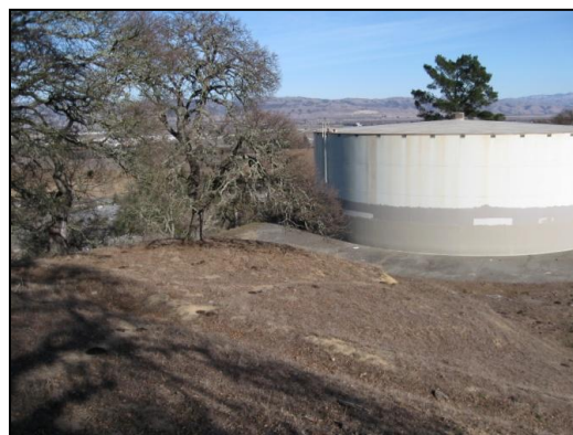
Photo 3: Existing Water Tank
